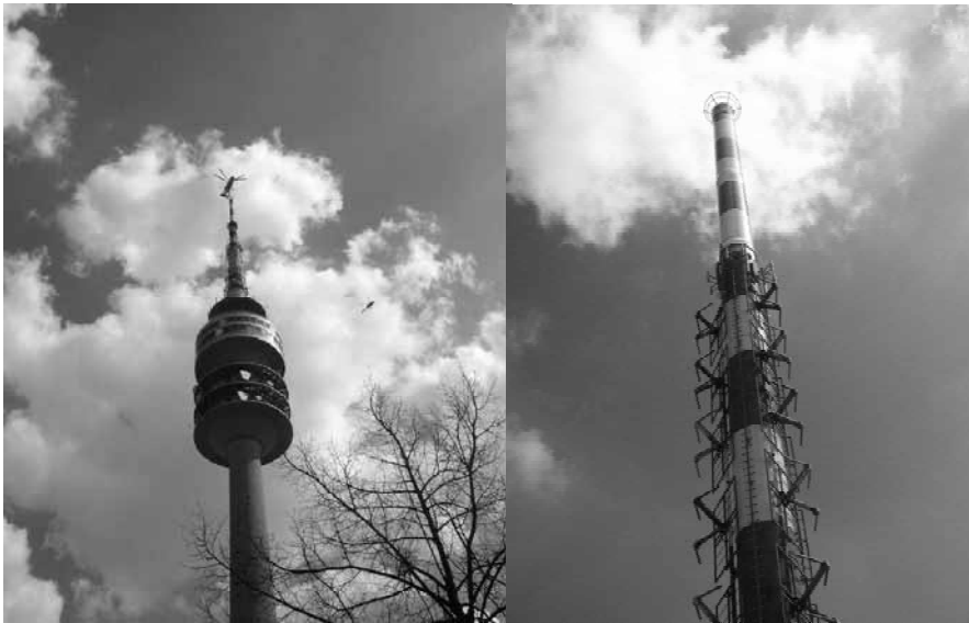
Fig. 31.17. Olympic Tower Munich; antenna installation for DVB-T using a helicopter (left) and Wendelstein antenna (right)
